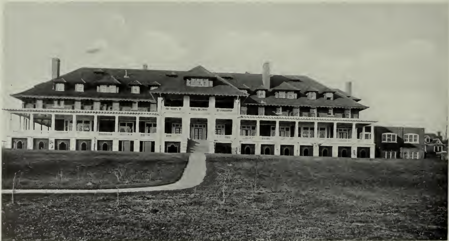
COUNTRY CLUB, DETROIT, MICH. ALBERT KAHN, ARCHITECT; ERNEST WILBY, ASSOCIATED.
